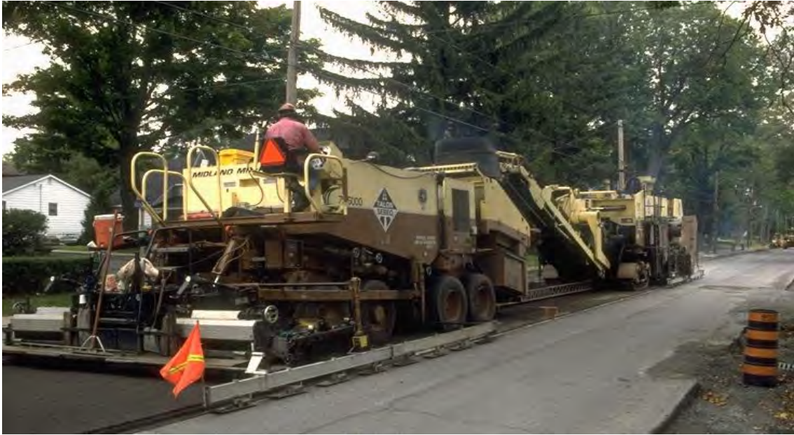
Photograph 3 - Two-unit recycling train
