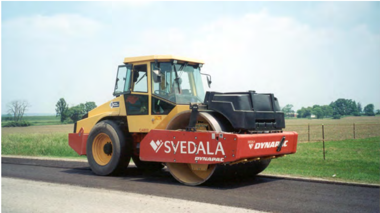
Photograph 8 – Modified large single drum vibratory roller fitted to compact cold recycled material
