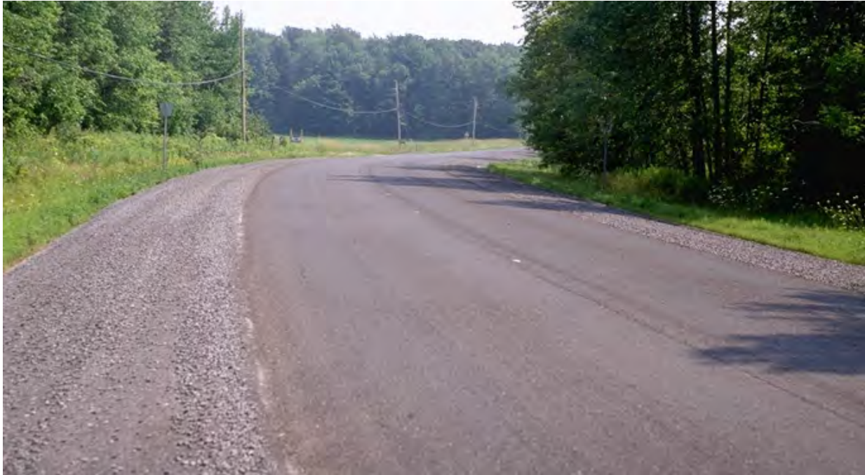
Photograph 10 – Rural Cold In-place Recycling mat prior to placement of wearing course
