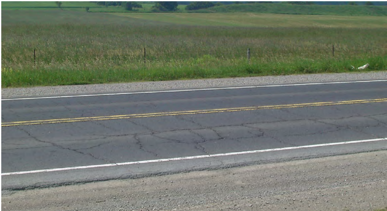
Photograph 1 – Well-drained structurally sound candidate for Cold In-place Recycling
