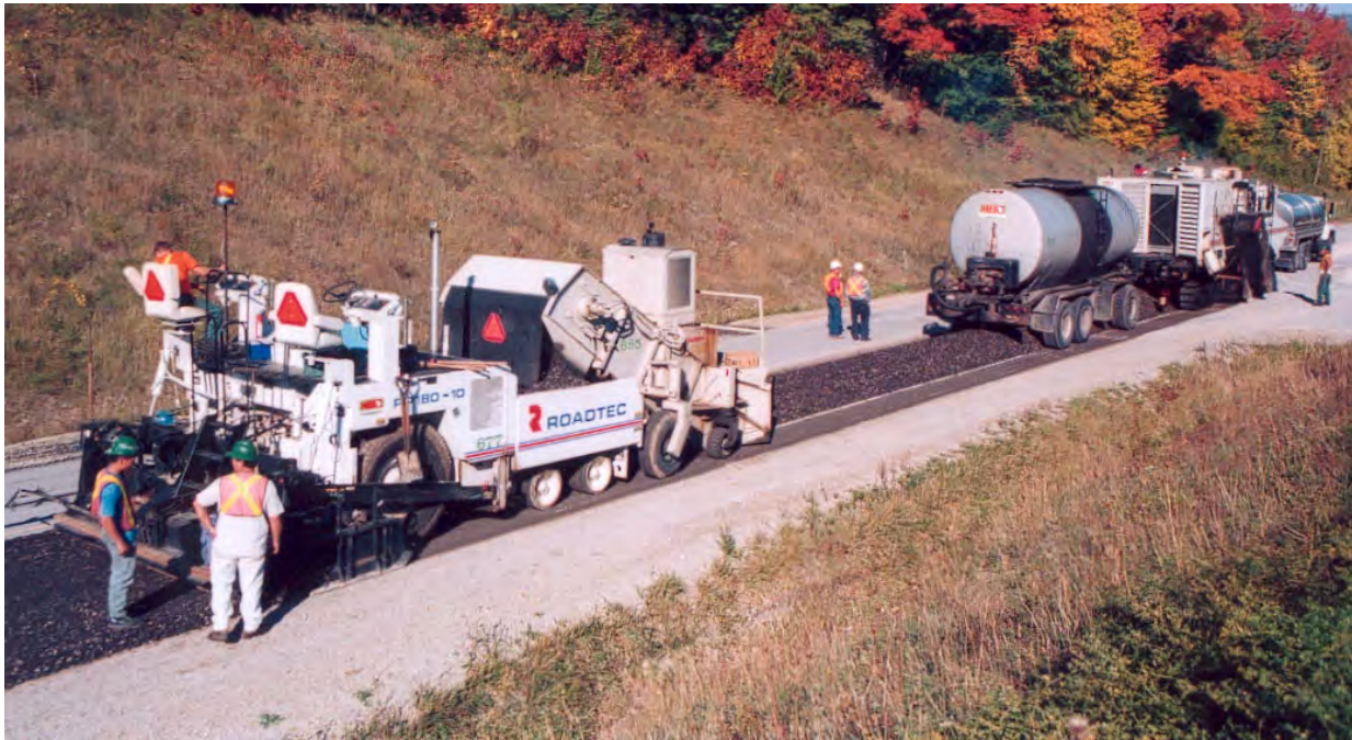
Photograph 2 - Single-unit recycling train with placement using a standard paver
